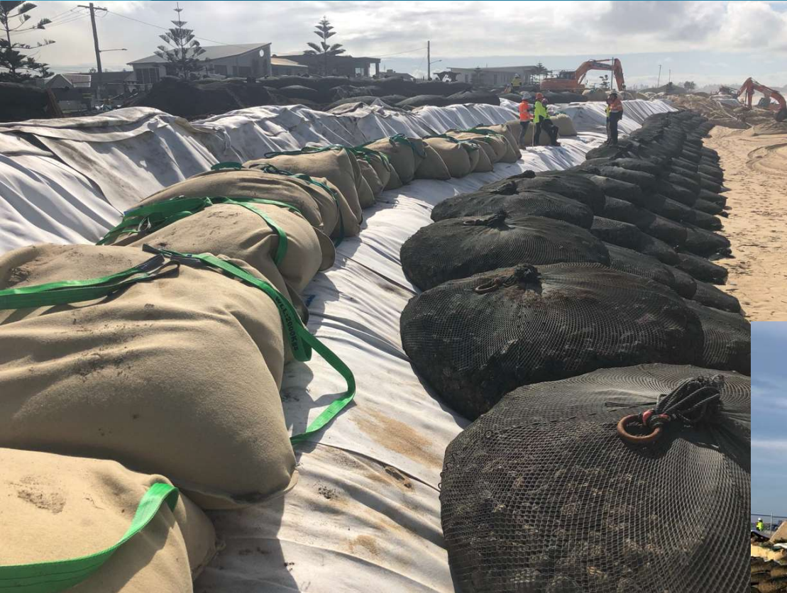
Articulating wrapped crest anchor
