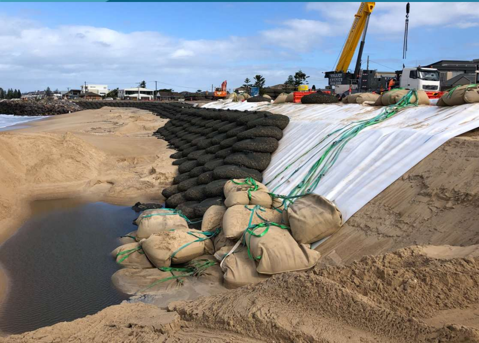
Daily protection and uncovering of leading edge of works
